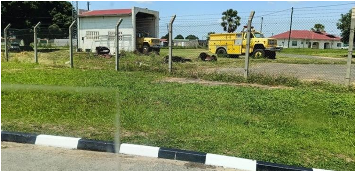
Figure 4: The only existing fire shade moreover outside the Aerodrome
