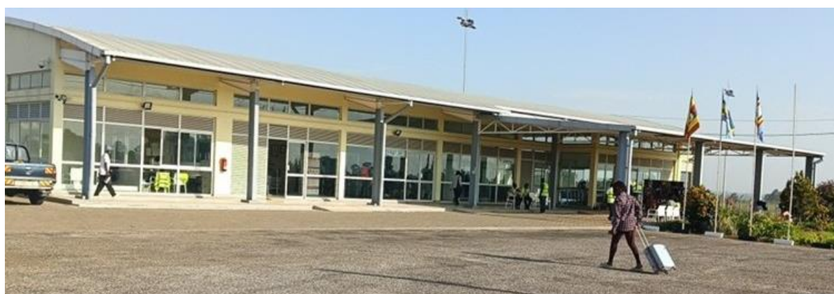
Figure 2: The recently constructed 200Pax terminal building
