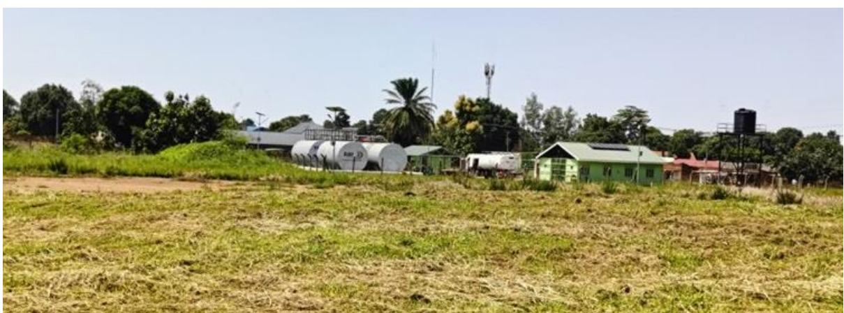
Figure 8: The temporary aviation fuel station
