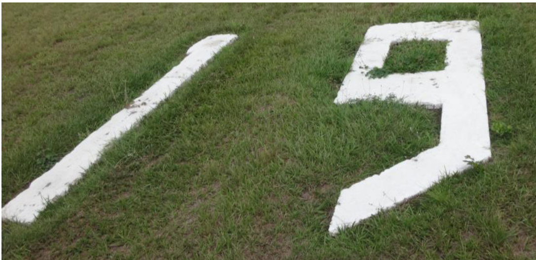
Figure 17: Example of runway designation marking in situ
