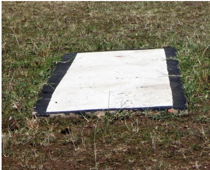
Figure 10: Example of a concrete runway edge marker
