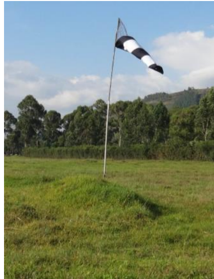
Figure 28: WDI mast bent and not marked
