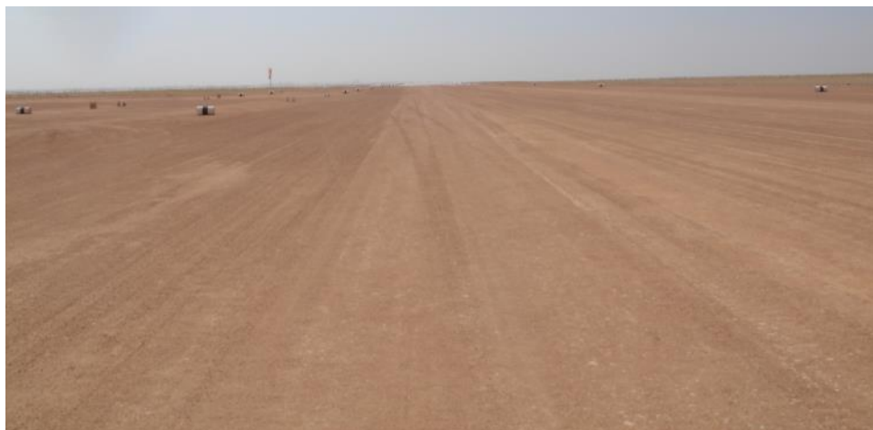
Figure 15: Sample: runway marked by black and white drums
